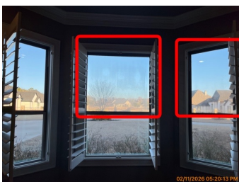
Downstairs front right bedroom
