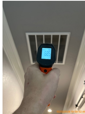
Downstairs main return
