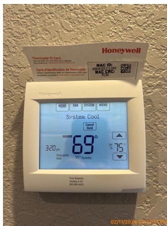
Downstairs front right Bedroom
