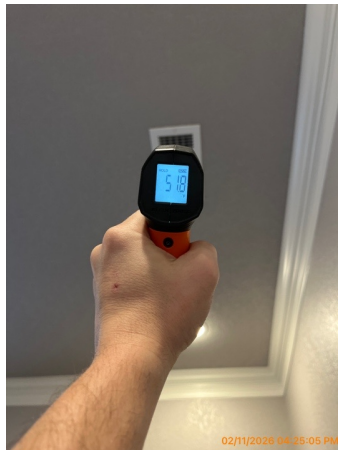
Downstairs back right bedroom supply
