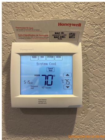
Downstairs front right Bedroom
