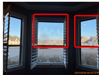
Downstairs front right bedroom
