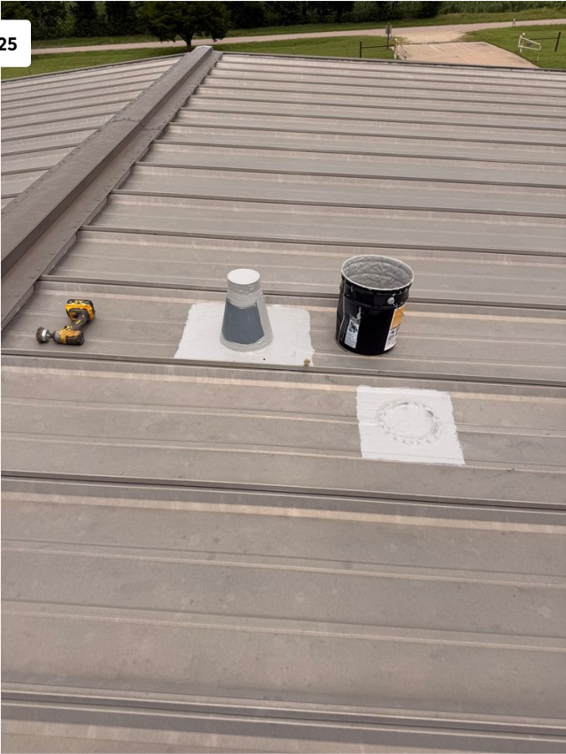
Project: 6415 W 95th St S Date: Jun 19, 2026, 12:46 PM Creator: Lucas Crump
