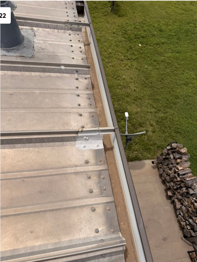
Project: 6415 W 95th St S Date: Jun 19, 2026, 12:29 PM Creator: Lucas Crump
