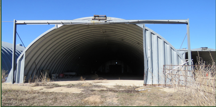
Quonset-Farm Utility Building
