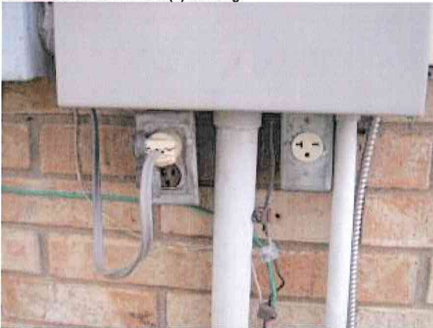
All exterior circuits should be GFCI protected with weatherproof covers/enclosures.
