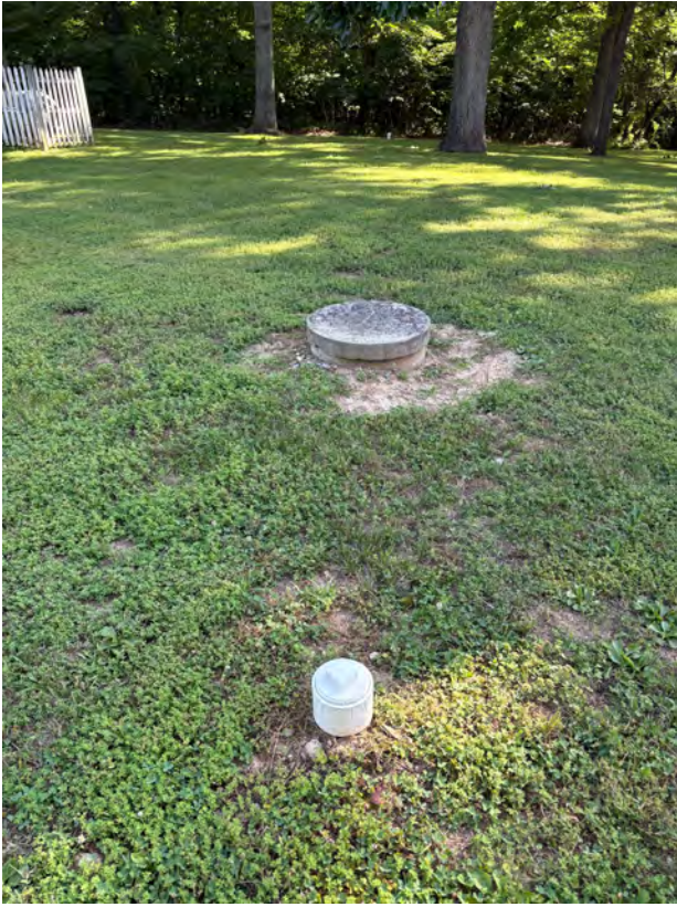
Clean out/ tank
